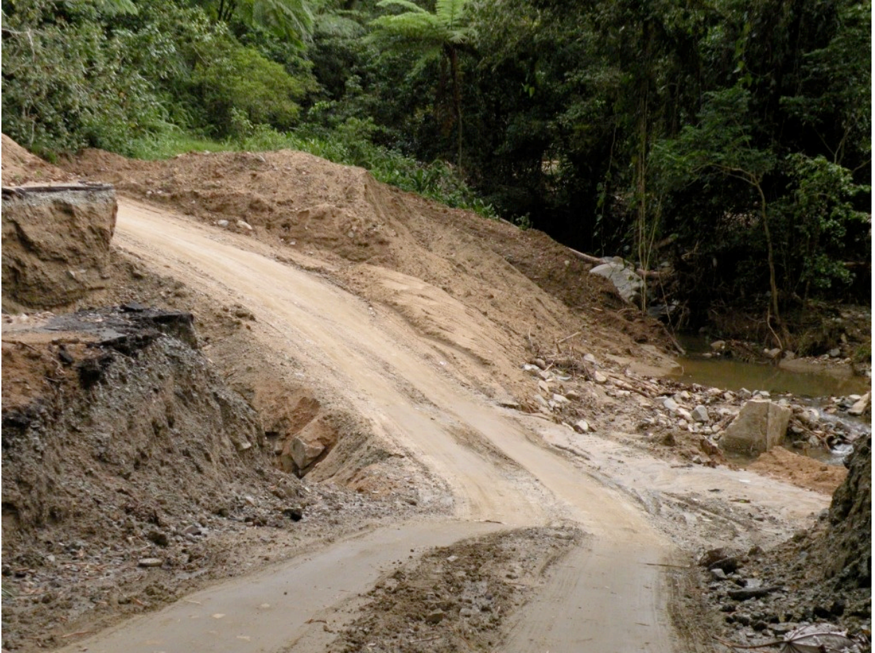
Roads collapsed in a locality where Eleutherodactylus cooki was present.
